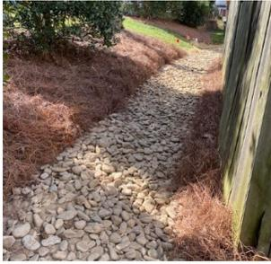
A French drain is a trench filled with gravel or rock, with or without a perforated pipe, used to redirect surface water and groundwater. This practice is a common means of diverting water from one location (ex. near a foundation or a wet area on a property) to another location (ex. municipal (City) storm drain or a nearby swale). A French drain diverts excess rainwater to dry soil that is excessively waterlogged.
